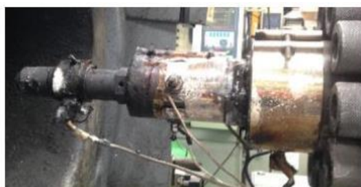
Partially enclosed heating
